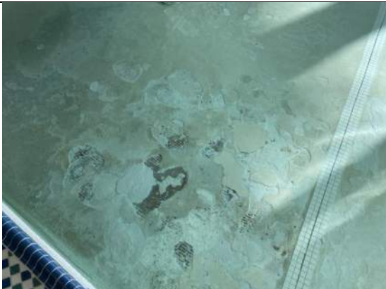
Figure 8 Plaster delamination
