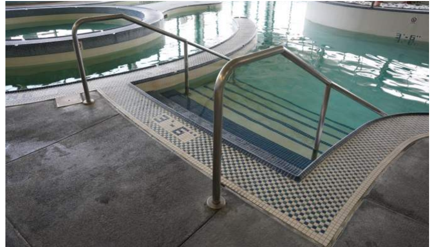
Expansion joint between colored concrete pool deck at perimeter pool tile band
