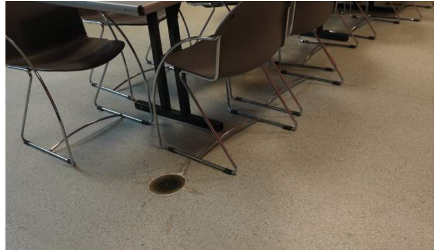
Patching of vinyl flooring at floor drain
