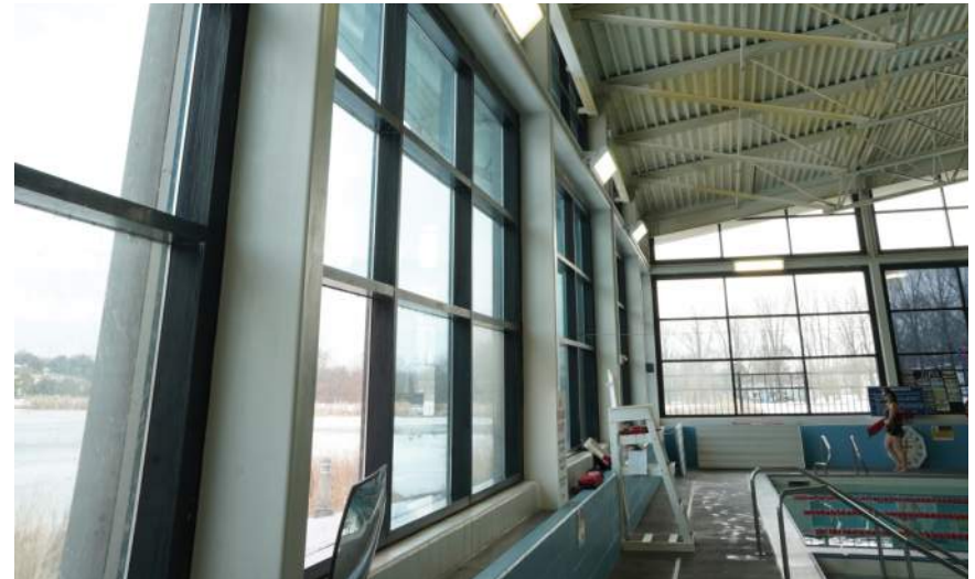
Exterior natatorium glazing and aluminum frame
