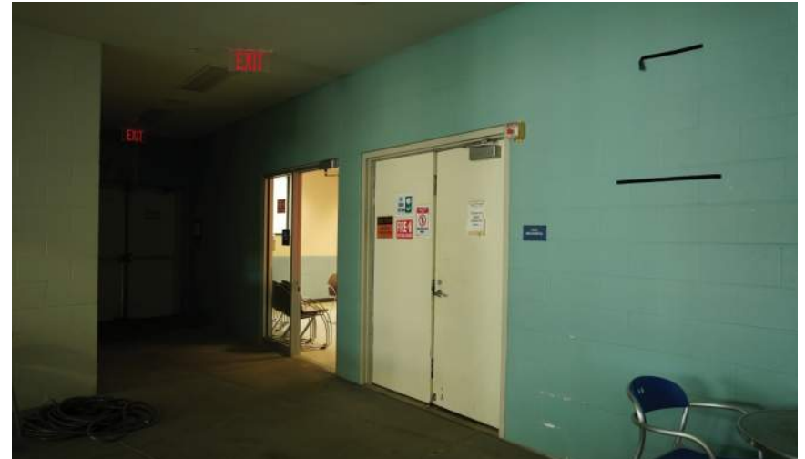
Access to Wet Multipurpose Room and Pump / Filter Room
